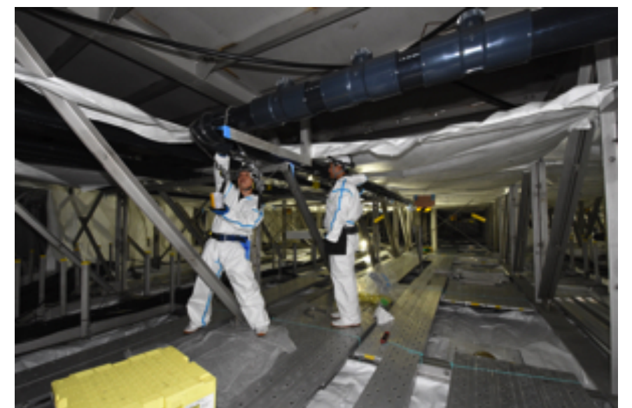
Install new water pipe
