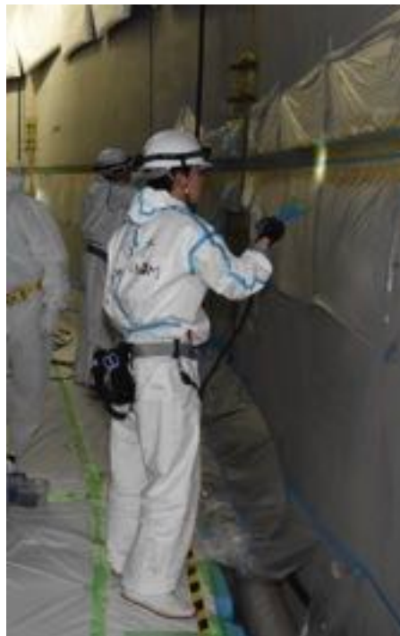
Seal whole welding lines
