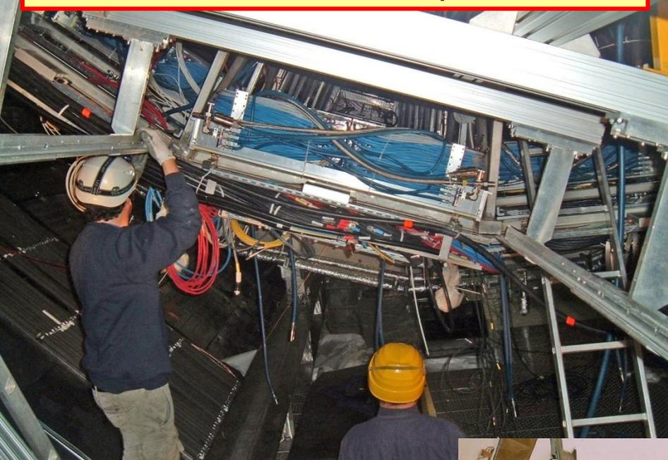
Installation of final muon chamber
